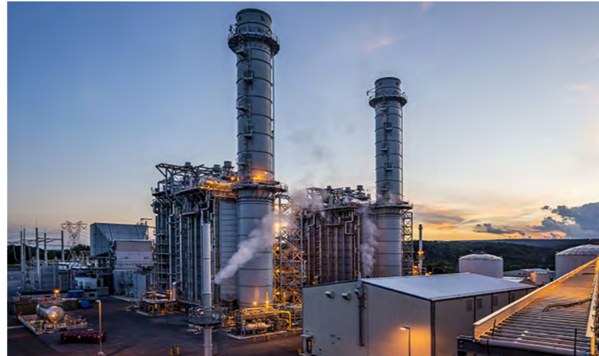
Fairview CCPP, USA
