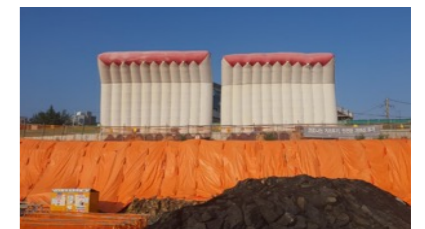
Installing protective barriers
