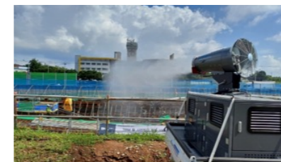
Using high-pressure water spray equipment
