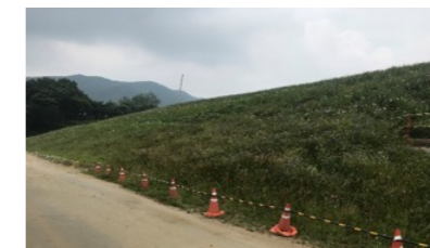
Greening embankment slopes
