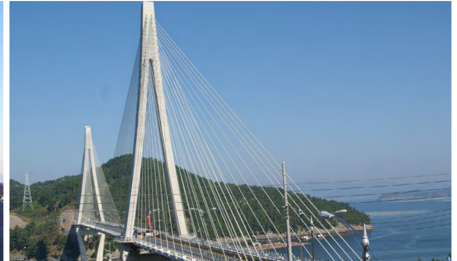
Saryangyeondogyo Bridge, Tongyeong-si, Gyeongsangnam-do
