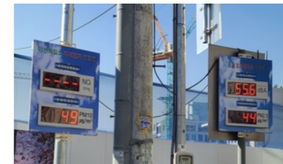
Installing particulate matter and hazardous substance status boards
