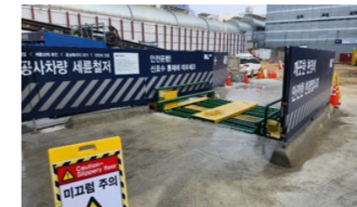
Operating wheel washing facilities
