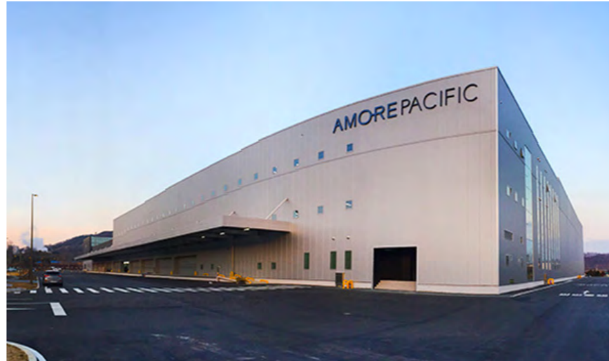
Amore Pacific's distribution center in Gimcheon
