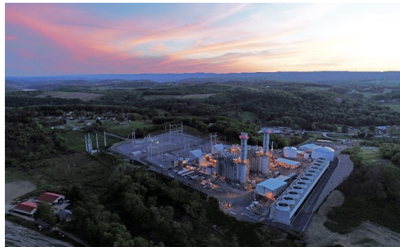
Fairview CCPP, USA
